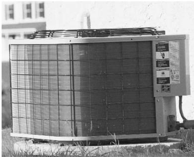
The condenser is the part of a central air conditioning system that discharges heat from your house to the outdoors.
