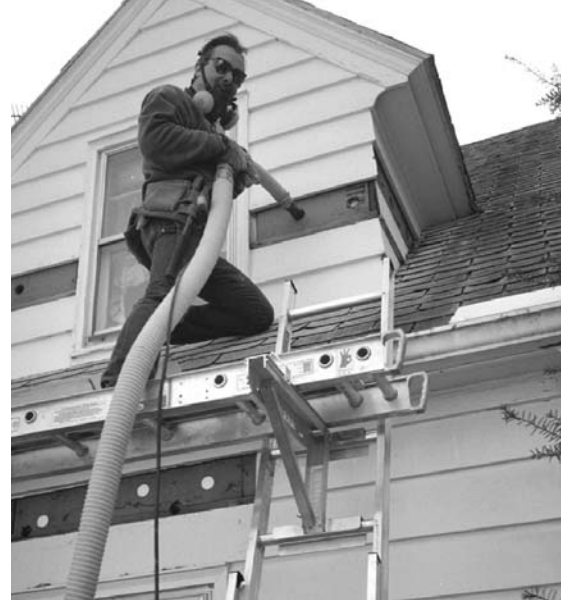
Installing blow-in insulation.
