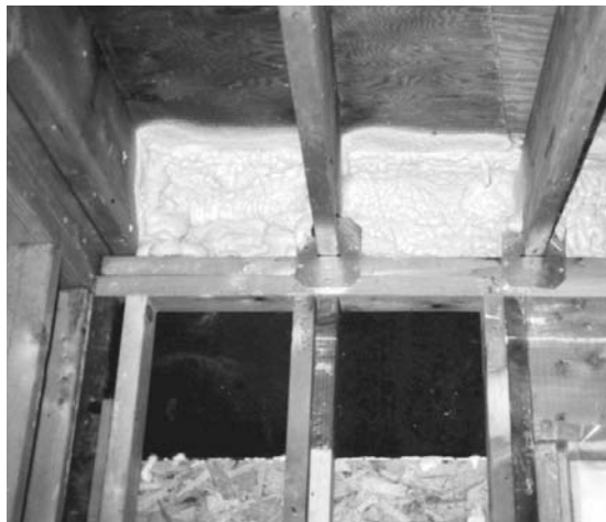
Insulating the sill box with spray-in foam.
